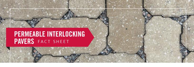
Permeable pavement systems have structural units that include void, or open, spaces, allowing stormwater to infiltrate and get treated and stored in an underlying gravel base. The stormwater is then filtered through native soils or is discharged through an underdrain. Permeable pavement systems include, permeable pavers (bricks or blocks), along with pervious concrete and porous asphalt. Permeable pavers use pervious void space located between the pavers that is
