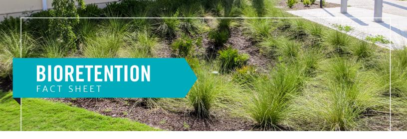
Bioretention is a shallow basin or landscaped depression designed to store, infiltrate and treat stormwater runoff. It is excavated and backfilled with well-draining, engineered soil media and planted with native vegetation, grasses or sod. Bioretention systems can also enhance habitat, mitigate for heat island effects and improve water quality.
