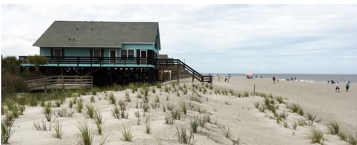
Figure 3. Beach-adjacent houses partly protected by beach nourishment and partial dune restoration on a South Carolina barrier island. Offshore sand was dredged and sluiced to the beach to replace sand lost to long-term erosion.
