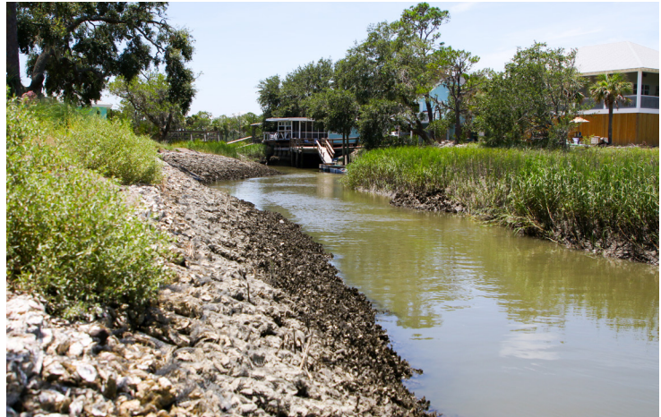
Figure 10. Living shoreline at the Burton 4-H Center on Tybee Island, GA. Courtesy of University of Georgia Marine Extension and Georgia Sea Grant.
