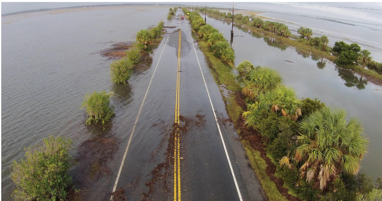
Figure 4. High tide flooding on U.S. 80, Chatham County, GA.
