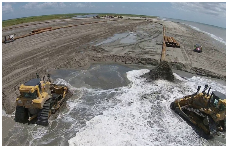
Figure 7. Spreading dredged sediments in a beach restoration project. Courtesy of USACE ERDC.
