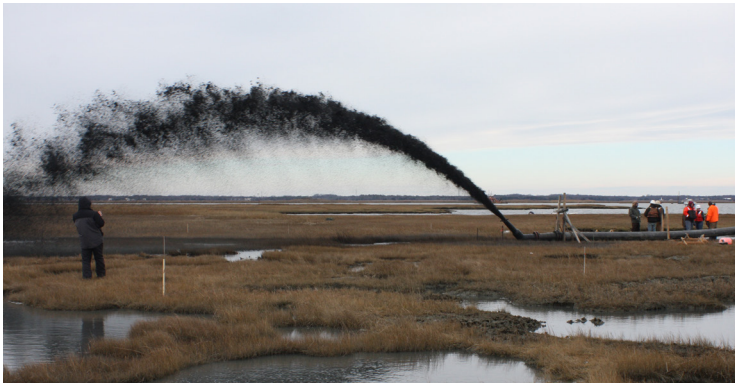
Figure 8. Thin-layer placement of dredged sediments to raise marsh elevations. Courtesy of USACE ERDC.
