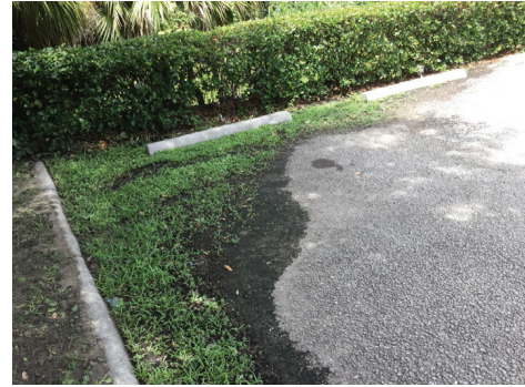
6 STANDING WATER, 12 VEGETATION (POOR) & 13 SEDIMENT (POOR)
