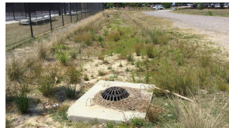
14 MULCH (NONE), 18 OUTLET DEBRIS, & 22 UNDESIRABLE VEGETATION (MARGINAL)
