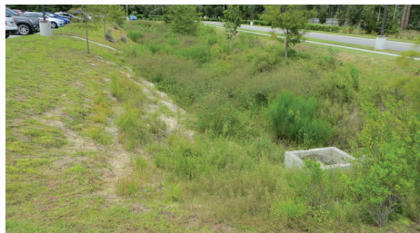
8 PRETREATMENT EROSION (SLIDE SLOPES) & 22 UNDESIRABLE VEGETATION (POOR)
