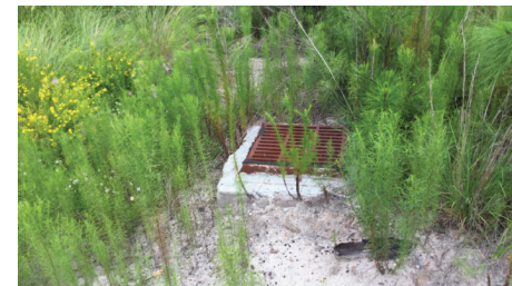
14 MULCH (NONE) & 22 UNDESIRABLE VEGETATION (POOR)
