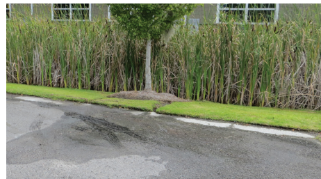
11 EXCESSIVE PONDING (CATTAILS & STAINING)
