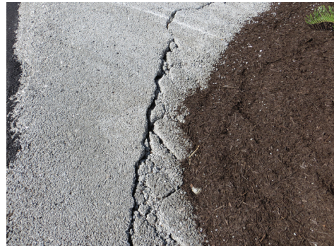
7 CRACKING-STRUCTURAL
