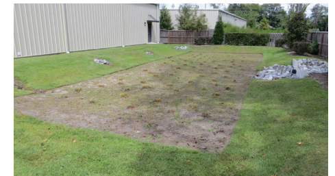
14 MULCH (NONE) & 24 PLANT DENSITY (POOR)
