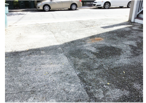
7 CRACKING-STRUCTURAL
