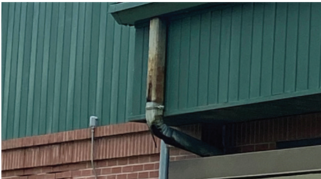
12 Gutters (Structural/Leaking)
