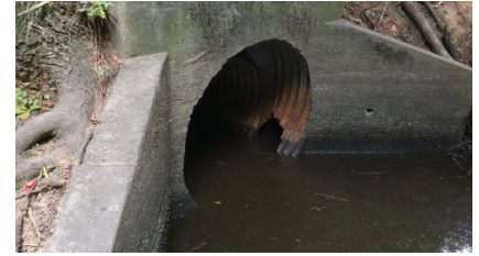
4 Pipe Corrosion
