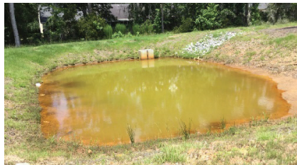
9/11 Sediment Stains & 10 Erosion
