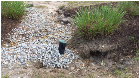
8 Inlet Erosion
