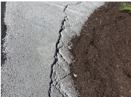
7 CRACKING-STRUCTURAL
