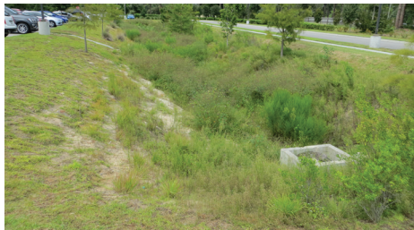
8 PRETREATMENT EROSION (SLIDE SLOPES) & 22 UNDESIRABLE VEGETATION (POOR)
