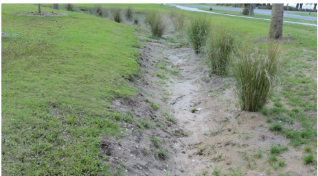
8 INLET EROSION (GRASS CHANNEL)
