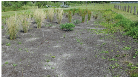
14 MULCH (<2''), 22 UNDESIRABLE VEGETATION (MARGINAL) & 24 PLANT DENSITY (MARGINAL)
