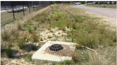
14 MULCH (NONE), 18 OUTLET DEBRIS, & 22 UNDESIRABLE VEGETATION (MARGINAL)
